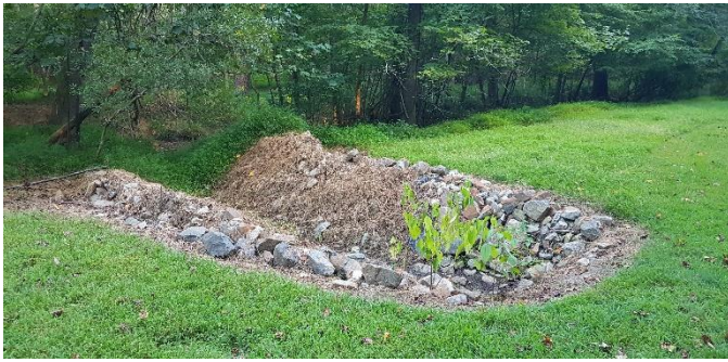
Figure 1. A detention pocket to enlarge the channel capacity on a piedmont tributary of a stream in North Carolina, USA (Photo by Yusuf Serengil).
